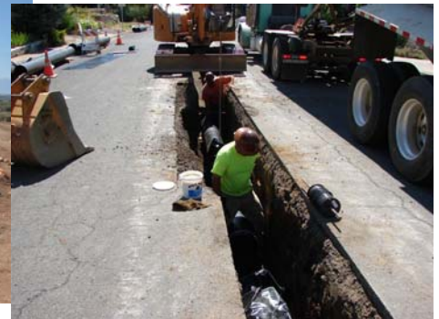
North Street Water Line
