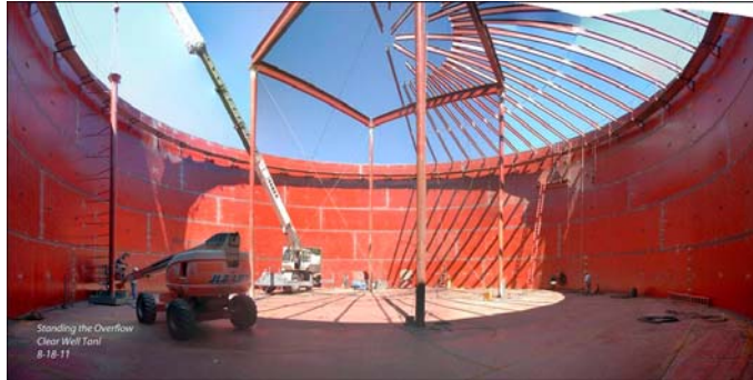
Crane raises the roof on the Clear Well Tank
