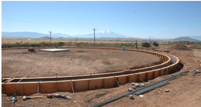
Ring Footing for Backwash Recycle Tank
