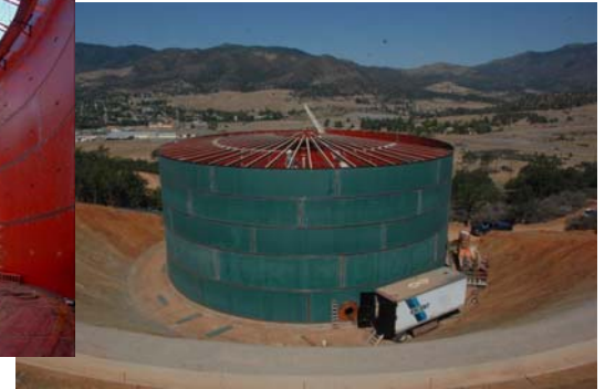
Upper View of the Clear Well Tank on Foothill Drive
