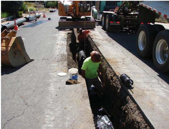
North Street Water Main replacement, August 29, 2011
