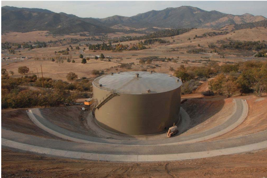
View on Butcher Hill looking down on the 2.5 million gallon Clearwell tank, January, 2012.
