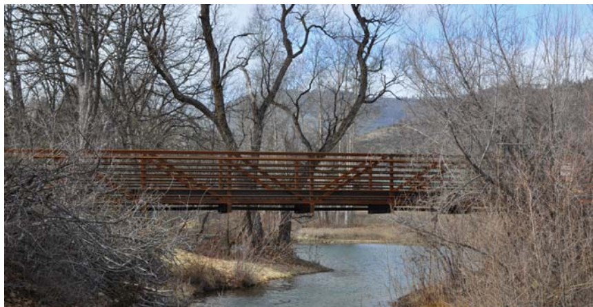
Greenhorn Park Pedestrian Bridge, February 2012
