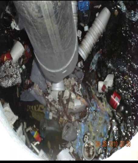
Debris in Center Street Trash Separator, 2010
